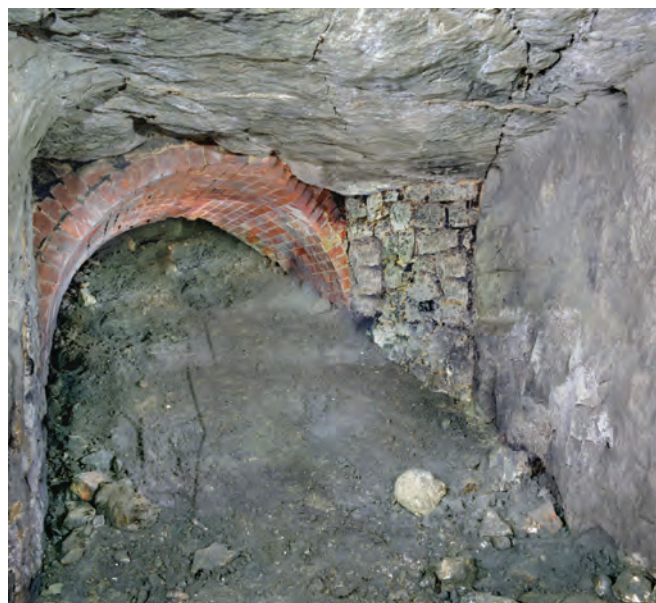
The brick arch is an original entrance, buried during the construction of the A22. Photo Nick Catford
